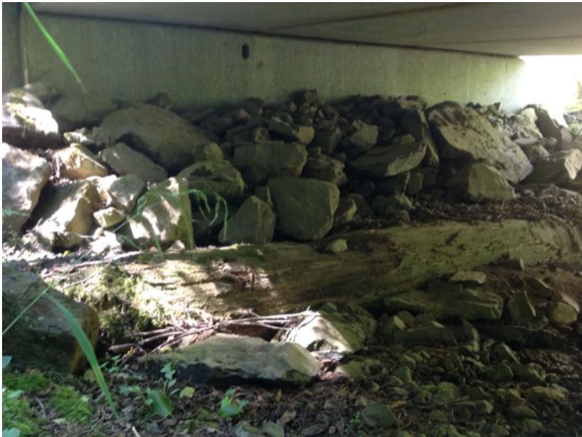
Left Bank Abutment when facing downstream
