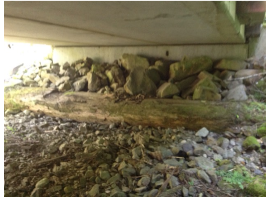
Right Bank Abutment when facing downstream
